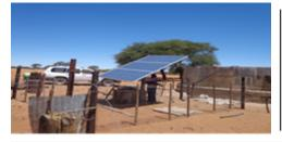
A Photovoltaic **Pumping System** produces energy for pumping water for livestock and domestic use.
